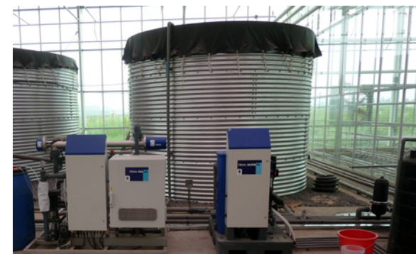
Figure 12. Standard dosing unit for drip irrigation (right) and UV disinfection unit (left).
