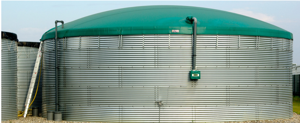
Figure 13. A tent construction film to cover the water basin.
